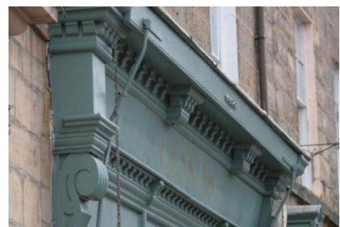
The fascia is protected and framed by the cornice. Sometimes the cornice seems to be supported by large brackets at each end, sometimes by small brackets (called dentils) that look like teeth. Sometimes by both, and sometimes by neither.
