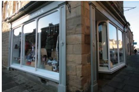
Mullions strengthen the glazed area, and limit the amount of glazing that needs to be replaced following a breakage.
